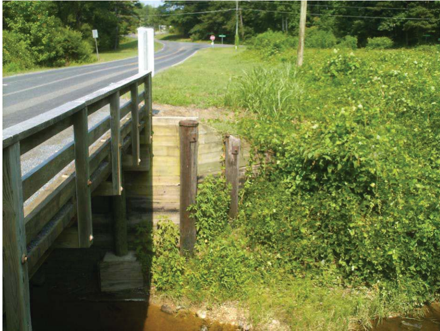
Photograph No. 5: View looking west at left side of End Bent 1
