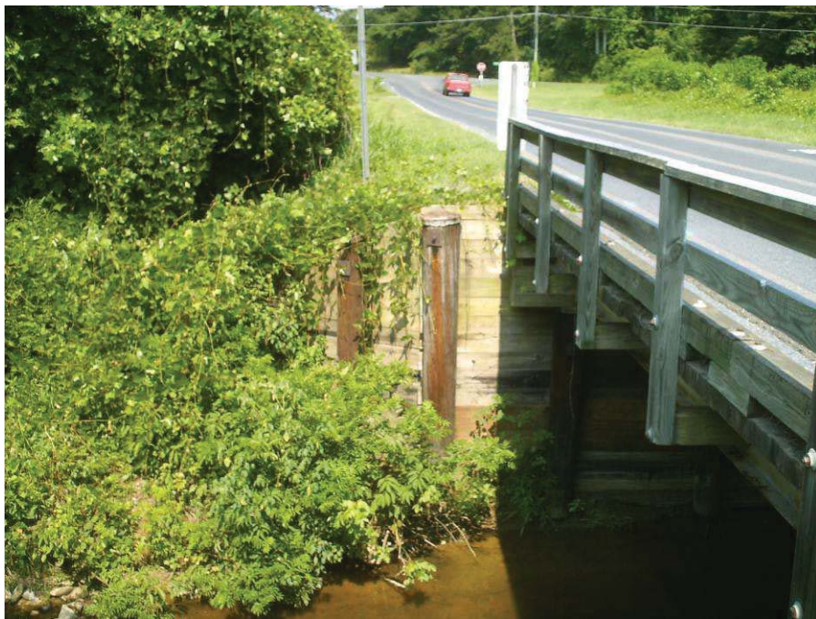
Photograph No. 6: View looking south at right side of End Bent 1
