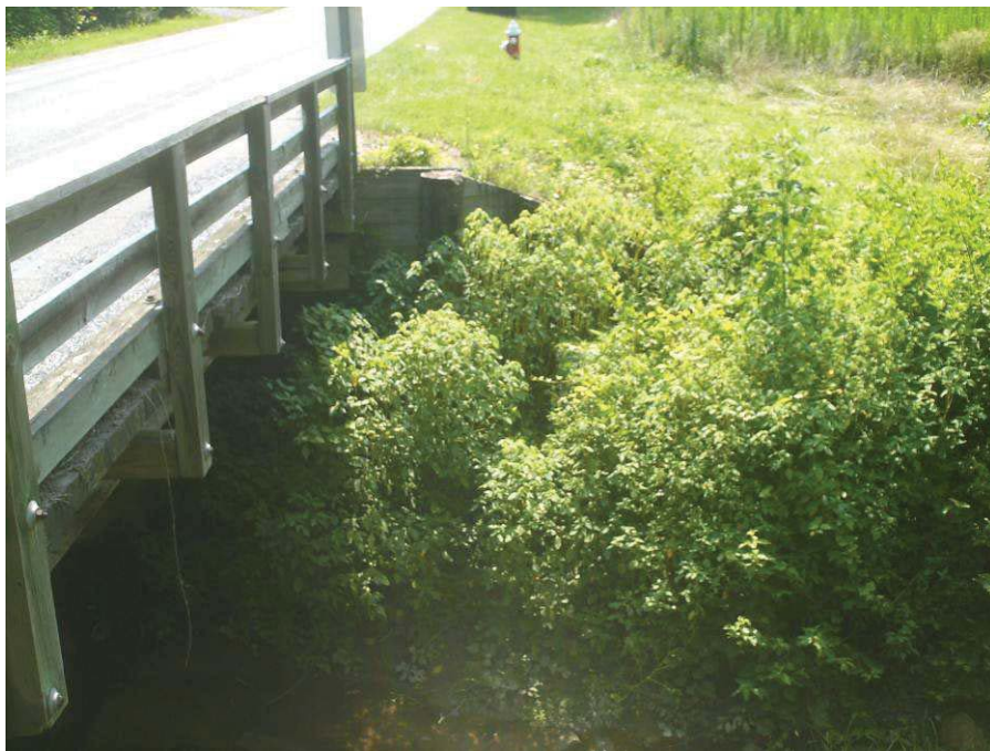
Photograph No. 8: View looking east at right side of End Bent 2
