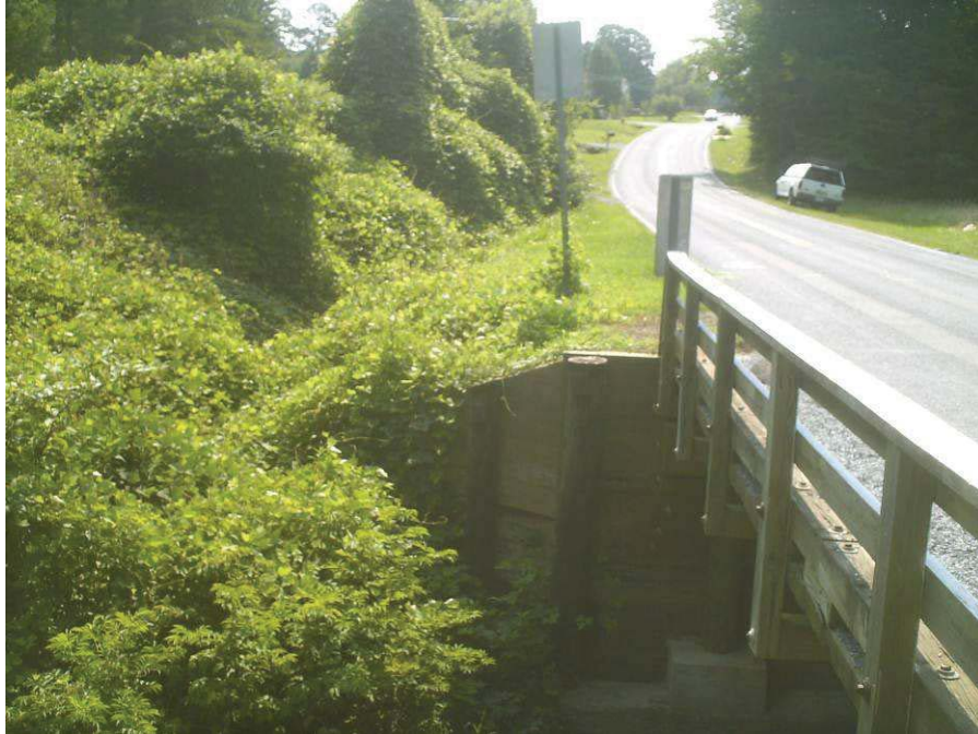
Photograph No. 7: View looking east at left side of End Bent 2
