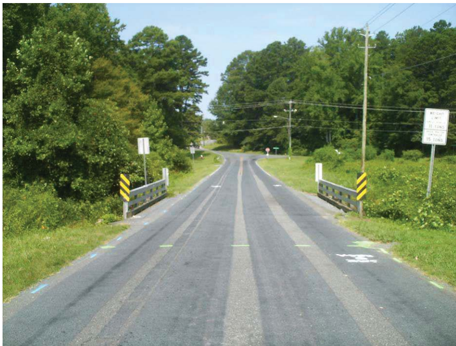
Photograph No. 2: View looking west down-station from east approach
